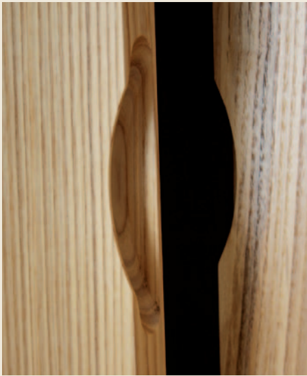
Recessed The handles are recessed into the edge, shaped with a drawer pull cutter
