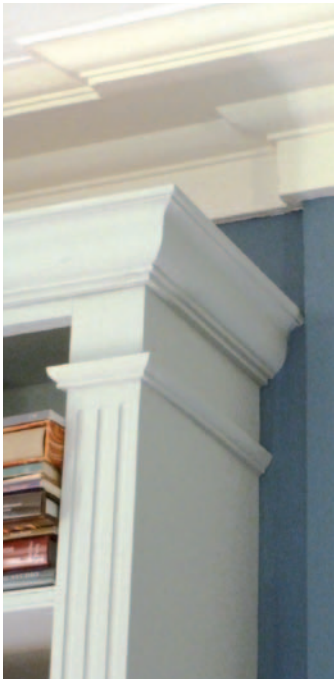
Pic.6 To create this short length of cornice, Gordon used a series of cutters. First he uses straight ones to form the three steps (or quirks). Then he removes as much of the waste as possible with straight cutters from the concave section until he has to use radius cutters to follow the curve. Then he planes away the convex section. It's a bit trial and error, but cheaper than getting cutters made
