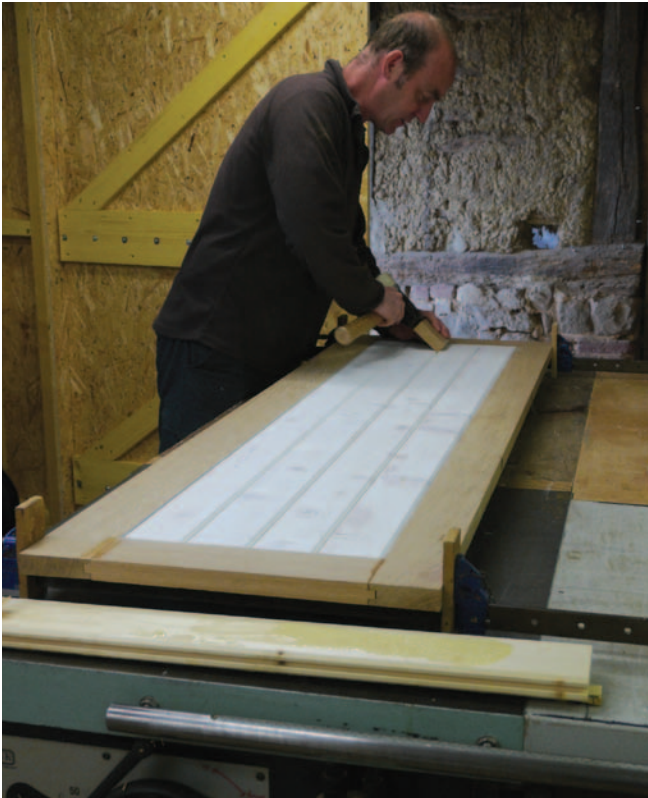
Pic.6 Testing the fit of of the T&G board. I use Rustins Knotting (rustins.eu). I always use it on softwood, where sap is the main enemy. All the shutters are to be painted, so I made sure to prime the tongues and grooves before assembly. I did not paint the tenons on the oak frames as these were to be glued
