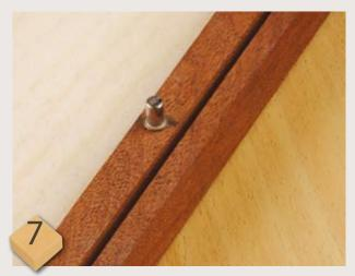
The polycarbonate sheet is cut to fit the slots and a ply shelf made that rests on small shelf supports fitted in the glazing bars. The whole cabinet needs to be sanded and a finish applied before the glazing is fitted
