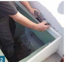
**3**The frame is an inverted U-shape because there cannot be frame at the bottom edge where the water runs off. Here a strap of oak *(Quercus robur)* is fitted underneath instead to maintain the frame integrity. The first job was to machine the glazing rebate with a big Wealden tenoning cutter.
