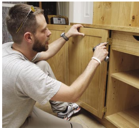
Hinged The doors are hinged with cranked hinges from Hafele. Steve loves the little Dremel driver for hinging
