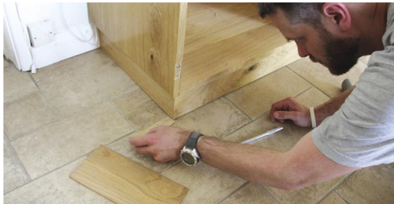
Fitting The top of the base unit is screwed to the supporting braces (D, left). Fortunately we had the compact drill/drivers on test at the time, and the Metabo was brilliant with its angled chuck. Steve used oak shims we'd produced when testing bandsaw fences a few issues ago
