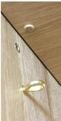
Details There are little leather locators on the underside of adjustable shelves (left) and wooden rests for the doors. The leather-covered magnets ensure gentle closing
