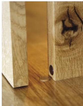
Details There are little leather locators on the underside of adjustable shelves (left) and wooden rests for the doors. The leather-covered magnets ensure gentle closing
