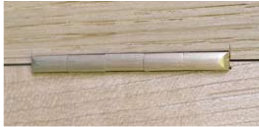
The hinge knuckle that protrudes can be softened by filing and rounding off
